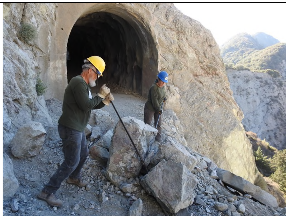
Guy Webster and Lauren Ballas removing boulders with rock bars at Mueller Tunnel. July 6, 2021.
